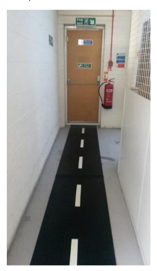
TELBAK Flexible black PVC matting is resistant to a wide range of chemicals (detailed list available on request); is resistant to attack by dilute acids at room temperature, although there may be some discolouration of the surface.
